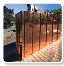
Architectural sheet metal has so many uses but it is most commonly used in custom fabrication of metal flashings, trim, and ornate metals used to create an architectural element on a building or home.
