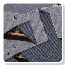
Steep-slope roofing is typically considered to be any roof system which has a slope equal to or greater than 3:12. These roof systems can be asphalt shingles, wood or cedar shakes, shingles, clay or concrete tile, or various metal or synthetic systems depending on decking, application and wind load.
